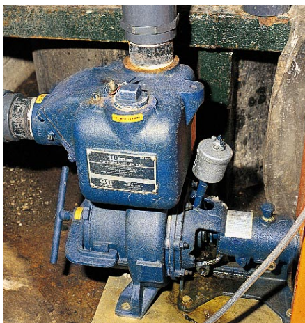
10 Series® pump transferring solids and corrosive liquids to a holding tank at a food processing plant in England.
